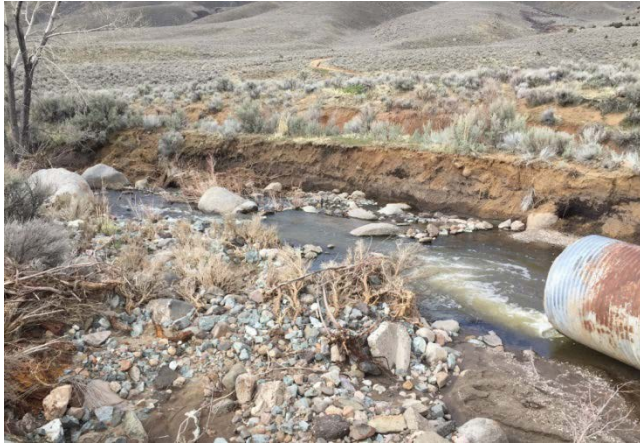
(L) Downstream damage to creek from washed out culvert; (R) Moon Rocks
